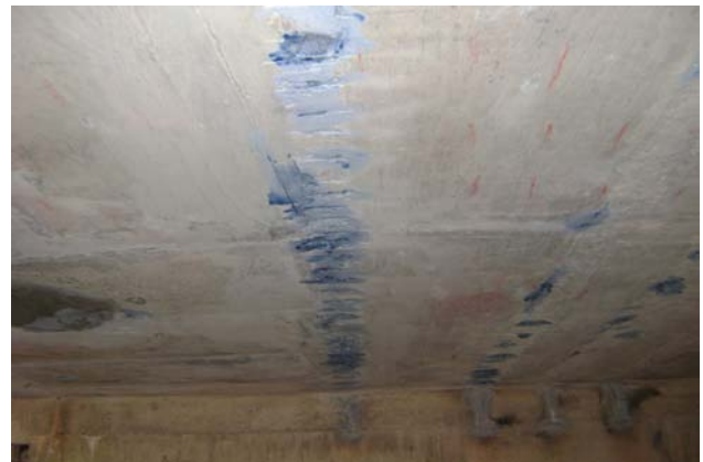
Figure 3 - Underside of Concrete Slab
