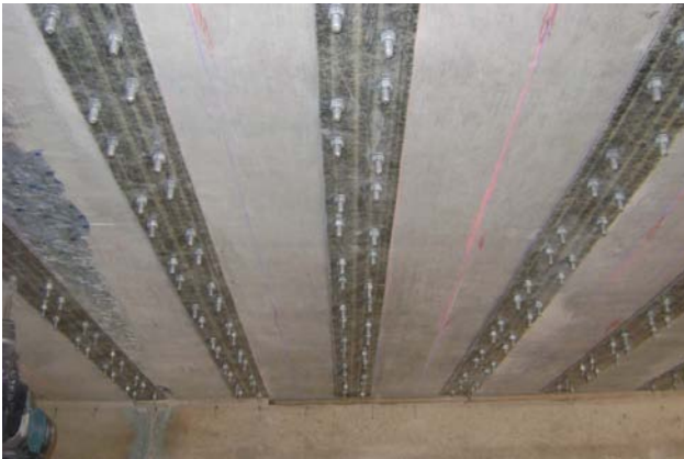
Figure 4 - Installed FRP Strips
