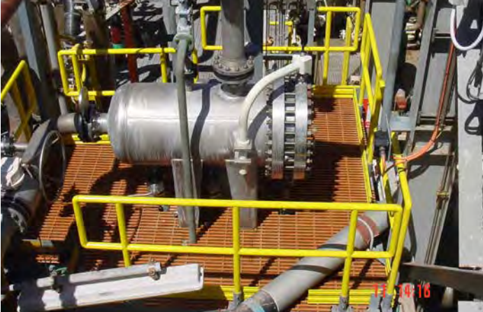
Separator Module Grating & Handrail DURAGRID® Phenolic grating and SAFRAIL™ handrail were used on this separator module.
