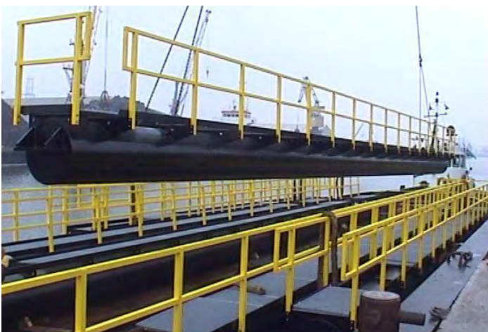
Floating ship access docks with low maintenance handrails.
