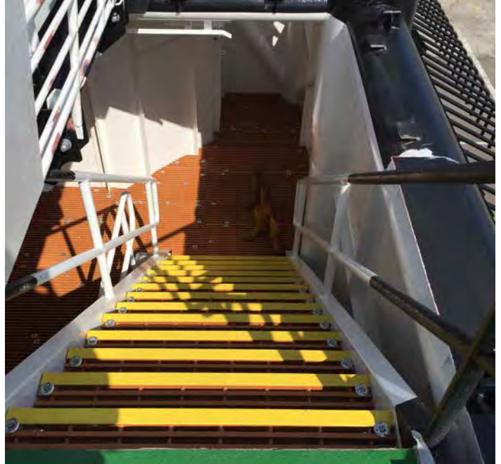
Separator Module Grating & Handrail DURAGRID® Phenolic grating and SAFRAIL™ handrail were used on this separator module.
