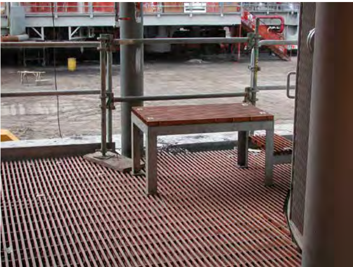
DURAGRID® Phenolic atop a small steel hop-up frame.
