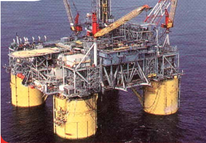
Largest use of FRP grating on an offshore platform at the time of its installation.
