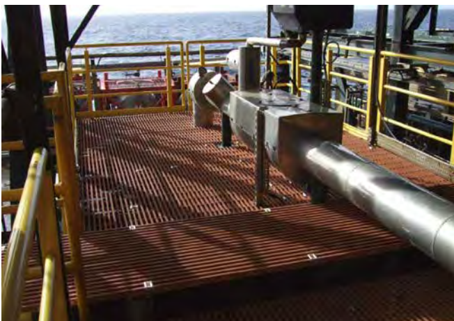
Starboard crane platform fully erected before being disassembled and shipped offshore.
