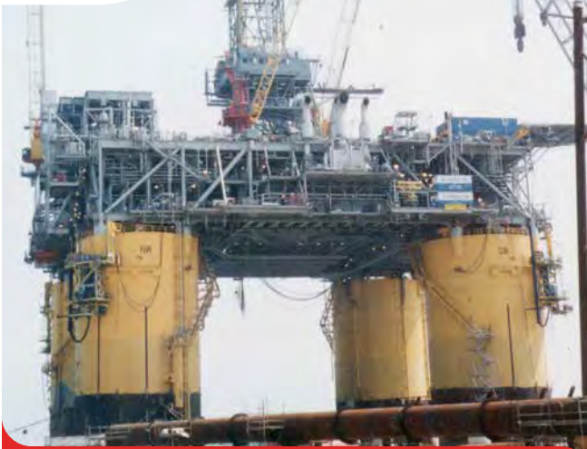
Largest use of FRP grating on an offshore platform at the time of its installation.
