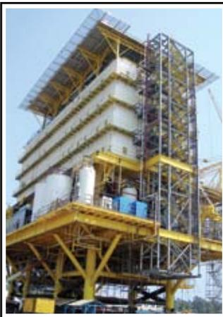
Both SAFRAIL™ and DURADEK® are pultruded with fire-retardant polyester resin and are low in thermal and electrical conductivity, key factors when considering the products were installed on the living quarter decks.
