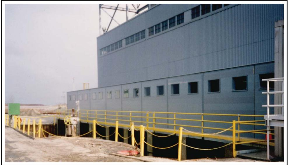
was a major factor that we had to consider. Also, the lightweight feature of fiberglass was important to us since we have to remove sections of the lean-to roof when we pull the screens up for maintenance. The insulation in the DURASHIELD® panels keeps the water from freezing and makes it much more comfortable for the workers, too."
