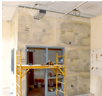
HS Armor under Drywall | Tennessee School Entry
