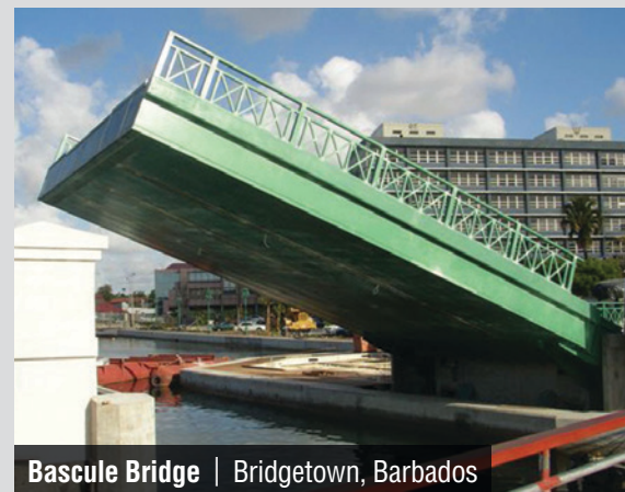
Fabrication of Above Bridge Bridge deck is constructed of both COMPOSOLITE® and COMPOSOLITE® HD
