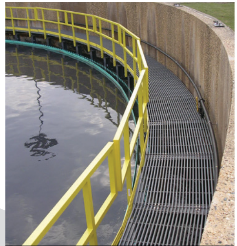
Water Treatment Plant | Albert Lea, MN
