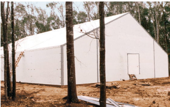
Compaq Computer chose a foam core panel building to assure RFI/EMI compliance for attenuation.
