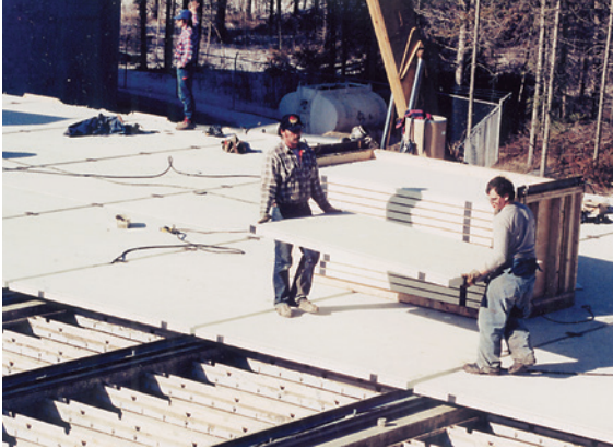
DURASHIELD® panels are used as plant roofs and chemical tank covers in corrosive environments, such as the covers (16,800 sq. ft.) (1,560 m 2 ) over anaerobic digester units pictured above.
