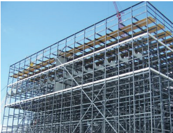
DURASHIELD HC® panels are commonly used in the construction of cooling tower interior partition walls.
