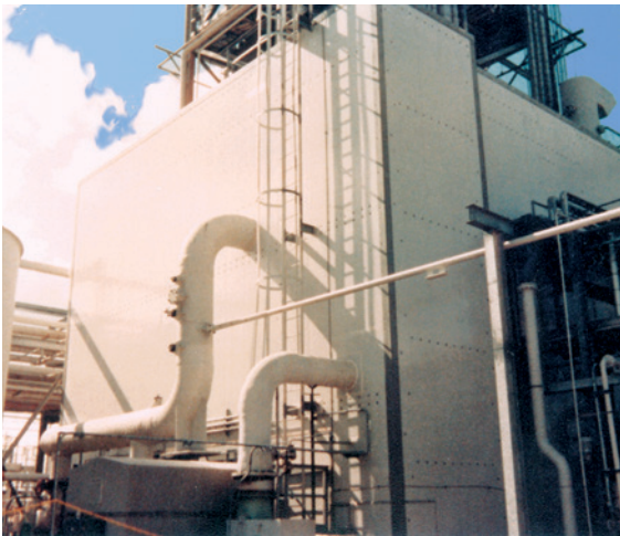
Airtight enclosure for Dow Chemical protects workers in adjacent areas against accidental escape of phosgene gas.
