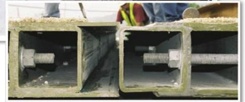
composite deck not only exceeds the life expectancy of the previous concrete deck but is also 70% lighter weight than a concrete deck. The deck allows the service load capacity of the bridge to be increased as well. The historic bridge will be completed by November 2006. ●
