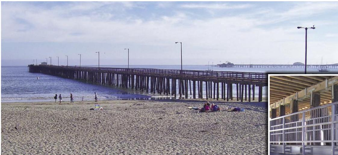
The Avila Beach Pier in California has been reconstructed using Strongwell's pultruded fiberglass structural materials. The 1,685-foot public pier was in need of a large stairwell at the end that would allow public access for landing boats and unloading guests.
