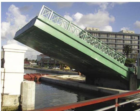
to-weight ratio of the pultruded parts. Heavier materials would have required the city to rebuild the lifting mechanism and other materials were not strong enough. The composite materials also offered the benefits of corrosion resistance, low maintenance and high aesthetic appeal.
