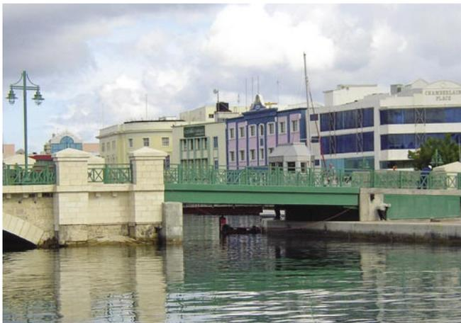
An all-composite double leaf bascule bridge recently installed in Bridgetown, Barbados, was built using Strongwell's COMPOSOLITE® building panel system, EXTREN® structural shapes and a custom heavy-duty building panel. The bridge superstructure itself is made entirely of COMPOSOLITE® system components and custom building panels, while various sizes of EXTREN® square tubes were used to create an attractive architectural railing system.
