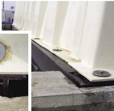
Thirty of the lightweight, double web beams were set into beam pockets in the concrete. The bottom flange of the beam was anchored to the concrete.
