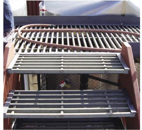
economical to ship and convenient to handle during installation. The fiberglass catwalk is also non-conductive and easy to maintain since the components will not require painting.
