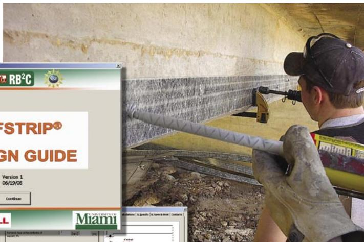
*The SAFSTRIP® Design Guide software is suitable for flexural analysis and design of simply supported reinforced concrete beams and one-way slabs strengthened with mechanically fastened FRP laminates subjected to uniformly distributed dead and live loads.*
