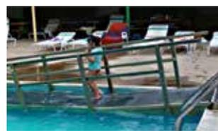
In addition to corrosion resistance, Strongwell's materials also provided valuable skid resistance. SAFDECK®'s fine grit surface provides a safe, skid-resistant walking surface in wet conditions.
