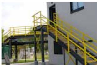
The Putnam Facility chose fiberglass versus galvanized metal because of the corrosive environment, reduction of labor, ease of installation, and low maintenance life cycle costs. GEF Incorporated fabricated the structure using EXTREN® fiberglass structural shapes, DURADEK® fiberglass grating, SAFRAIL™ Handrail, and SAFRAIL™ Ladder and Cage products.
