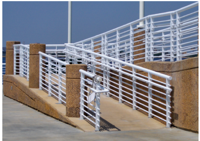
The Moody Gardens Theme Park has embraced the low maintenance and corrosion resistance of Strongwell's custom fiberglass railing systems. A day dock at the popular destination features an ADA compliant custom handrail system that uses several of Strongwell's pultruded fiberglass structural profiles.
