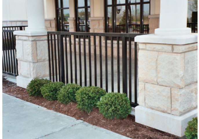
A custom guardrail system installed for Karlo's Bistro blends with surrounding architecture and adds aesthetic appeal.
