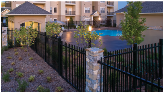
Rupe Building Co. installed Strongwell's maintenance-free fiberglass fencing (foreground) & guardrail (background) for this apartment complex in Oklahoma. The fencing mimics the "wrought iron look" without rusting worries.
