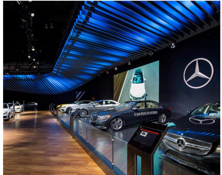
The team at Dimensional Communications Inc. wrestled with the European design, ultimately deciding weight and durability could be achieved by using Strongwell's pultruded FRP at custom lengths ranging from 4 to 20 feet. Each custom FRP component measured 16 inches in height and 2 inches in thickness.
