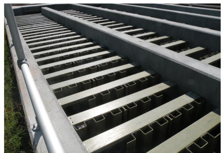
Engineers have begun to utilize lightweight FRP baffle panels for underwater flow control applications. In addition, the longer life cycle of the FRP and new design systems give engineers great flexibility in both new and retrofit projects for aeration chambers, contact chambers, and retention basins. ●
