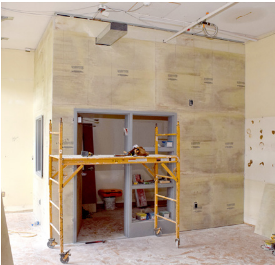
HS Armor can be finished to imitate drywall, as was done in the waiting area of this municipal building.
