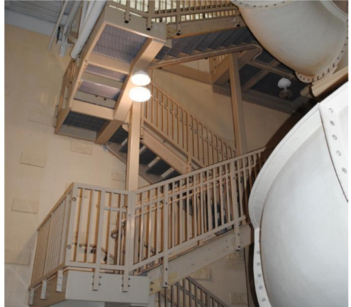
able to fabricate DURAGRID® I-4000 pultruded grating and stair treads, STRONGRAIL® handrail and multiple EXTREN® Series 625 structural shapes onsite without the use of welding or dangerous heavy machinery.
