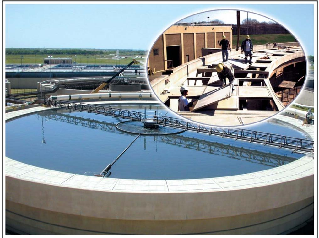
"Using fiberglass allowed the workers to be able to walk on the cover without it getting too hot. The doors in the covers were also large enough so that a person could get into the trough for cleaning and maintenance," Lindsay said. "There is a big potential in this market for this application."
