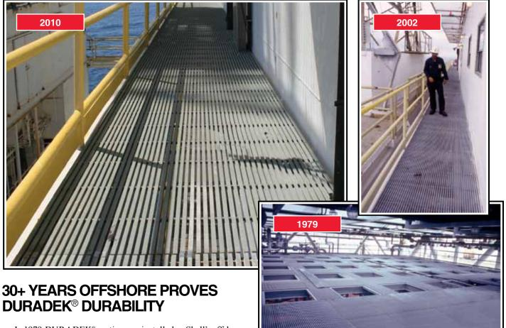
In 1979, DUR ADEK® grating was installed on Shell's offshore platform Ellen. The platform was destined for the Beta Field off the shore of southern California. Now, with over 30 years of use, the nearly 10,000 square feet of grating continues to show an excellent return on investment for current operators, Beta Offshore.
