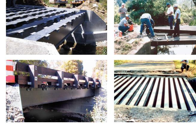
**Above:** The 36" x 18" EXTREN DWB<sup>®</sup> was installed in a Federal Highway Administration (FHWA) sponsored demonstration bridge project as part of the Innovative Bridge Research and Construction Program (IBRC) in September 2001. University professors from Virginia Tech performed a series of tests on the 36" x 18" EXTREN DWB<sup>®</sup> including stiffness testing of each beam. Eight beams were selected for the 38' span AASHTO HS-20 bridge located on Route 601 in Sugar Grove, Virginia.
