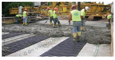
**Above:** A bridge on US Highway 12 over Coffee Creek in Black River Falls, Wisconsin required 2,400 sq.ft. of FRP deck form. Strongwell supplied 12" x 42" sections of SAFPLANK<sup>®</sup> with grit applied between the flanges. SAFPLANK<sup>®</sup> panels rested flange side up on a 3-1/2" x 1-1/2" ledge along both sides of the 54W pre-stressed girders, creating a clear span of 36". This installation eliminated the need to form between the girders and remove the forms after concrete was placed.
