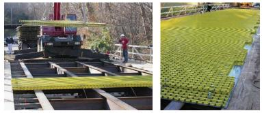
This field application in Greene County, Missouri, shows the GRIDFORM™ installation from start to completion. As you can see, FRP panel setting, anchoring and concrete forming is easily done with a small work crew. The 144-foot bridge deck and concrete railing system was completed in just five days.
