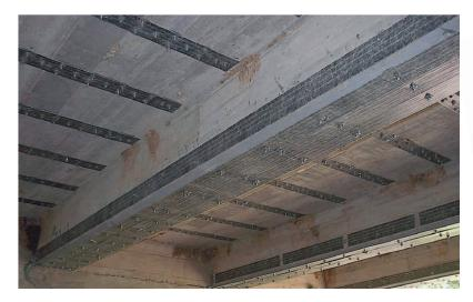
**Above:** The posted load for this bridge that spans the Meramec River in Missouri was increased from 10 tons to 18 tons by installing SAFSTRIP<sup>®</sup> using the mechanically fastened FRP system.
