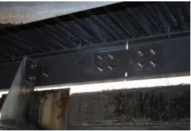
**Above:** A walkway spanning over a creek in Franklin County, Ohio, needed to be refurbished when heavy exposure from vehicular runoff rusted the existing steel. The walkway was rebuilt using corrosion resistant SAFPLANK<sup>®</sup> along with EXTREN<sup>®</sup> structural supports.
