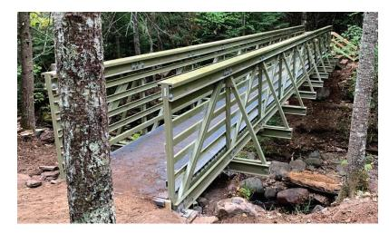
**Above:** This 50' long, 4' wide trial bridge installed near Gran Marais, MN, was designed using EXTREN<sup>®</sup> series 500 structural shapes and SAFPLANK<sup>®</sup> interlocking decking panels with a nonskid coating, which is capable of handling up to 90 PSF for live pedestrian loads.
