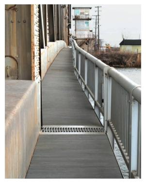
**Above:** The Cleveland Lift Bridge in Cleveland, Ohio utilized DURADEK<sup>®</sup> T-5000 (now DURAGRID<sup>®</sup>) pultruded grating to replace metal pedestrian walking surface which had rusted away.
