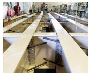
Left & Above: A golf course in the Cayman Islands needed a dual-purpose bridge at their facility to support golf cart traffic and allow watercraft to pass below. EXTREN<sup>®</sup> structural shapes, FIBREBOLT<sup>®</sup> threaded studs and nuts, and DURAGRATE<sup>®</sup> molded grating combined for a lightweight, corrosion resistant, and attractive solution for this 38' long, 10' wide single-leaf retractable bascule bridge.
