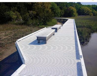
**Above:** This 400' walking trail boardwalk extension off the coast of South Carolina was recently rebuilt using EXTREN<sup>®</sup> structural shapes and DURAGRID<sup>®</sup> T-1800 pultruded grating after the old wooden structure did not withstand a hurricane.
