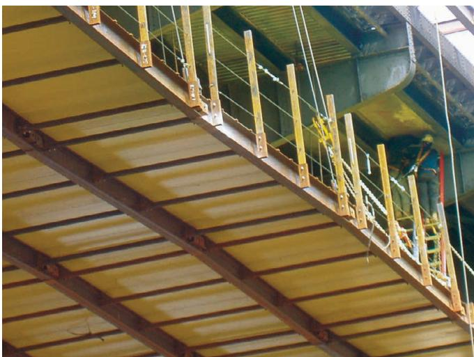
COMPOSOLITE® building panels are incorporated into reusable scaffolding in this bridge reconstruction project. The panels were pultruded in a safety yellow color and served as working platforms when construction workers replaced the bridge's bearings. Upon completion, the panels can be stored for use on future projects.
