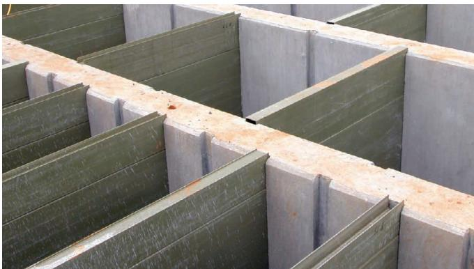
Versatile COMPOSOLITE® panels serve as a baffle system in this chlorine contact chamber.
