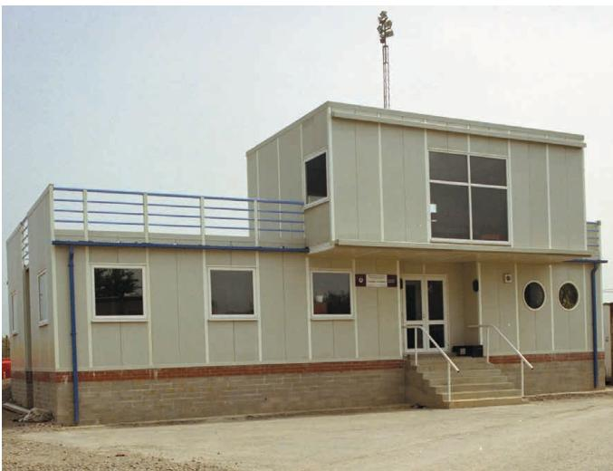
A visitor center in Bristol, UK, is constructed of COMPOSOLITE® panels, 3-way connectors, and toggles with no supporting frame. Cells of panels and 3-way connectors were filled with foam for thermal insulation.
