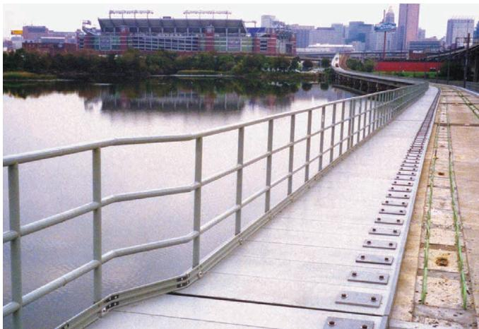
COMPOSOLITE® panels and SAFRAIL™ handrail compose this walkway installed along a commuter rail track by the Maryland Transit Administration. The nonconductive and corrosion resistant FRP walkway provides a safe walking surface and has lower installation and maintenance costs than a steel walkway.
