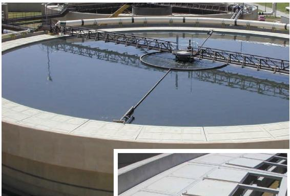
Odor control covers at the Trinity River Waste Water Treatment Plant in Dallas, Texas, utilize COMPOSOLITE® panels because of the product's extensive benefits. The panels provided strong, lightweight, corrosion resistant covers for the large wastewater treatment facility.
