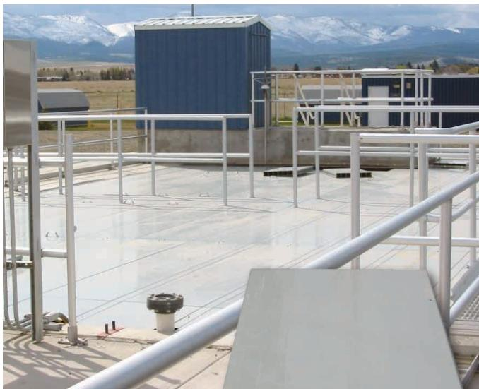
COMPOSOLITE® panels are ideal for use as odor control covers. The strong yet lightweight covers are easy to handle and can withstand the harsh environment for years. The panels also require little to no maintenance.
