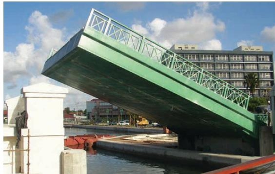
An all-composite bascule bridge in Bridgetown, Barbados, was built using Strongwell's COMPOSOLITE® building panel system, COMPOSOLITE® HD heavy-duty building panels, and EXTREN® structural shapes (see assembly in-process photo below). The drawbridge is mainly used by pedestrians in this tourist destination.
