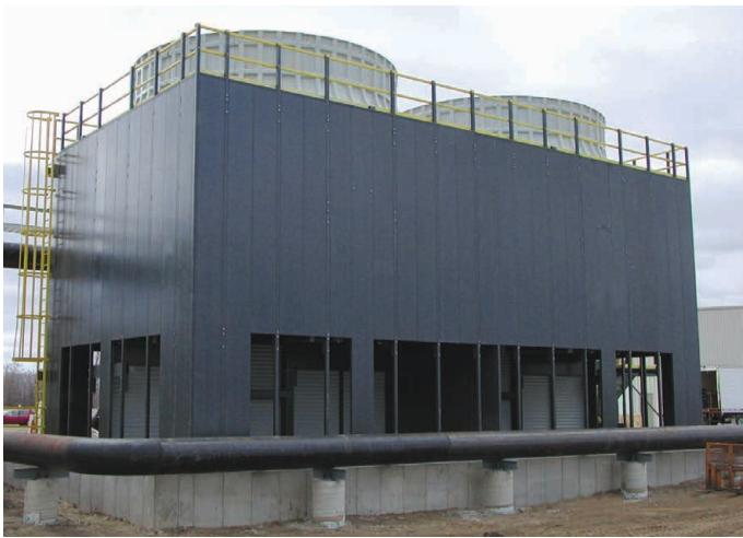
COMPOSOLITE® panels withstand the harsh environment of cooling towers with ease. The panel system not only provides excellent structural properties, but the rot and corrosion resistant panels will last for years to come.
