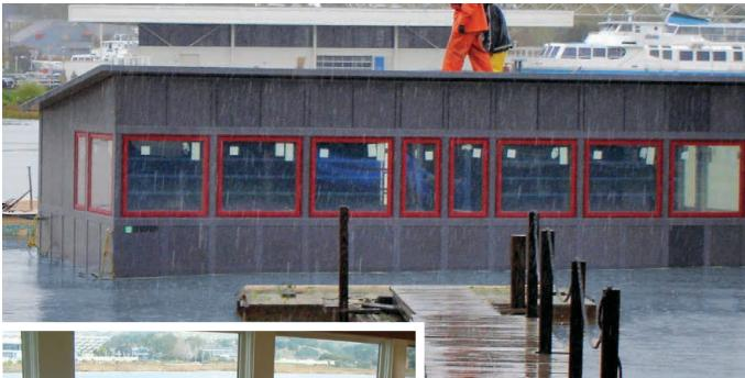
A floating office in the San Francisco Bay was constructed using the COMPOSOLITE® building panel system. The fiberglass structure was designed using COMPOSOLITE® FRP panels because they are less expensive than steel or concrete and were also easy to assemble.
