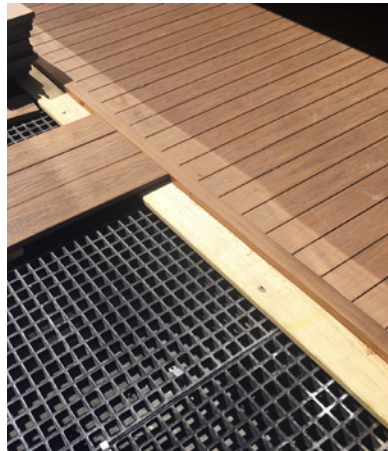
This New York City, NY housing development used DURAGRATE® as subflooring material for their rooftop space. The landscape architect needed a lightweight, bi-directional load, subflooring product which could be easily fabricated onsite.
