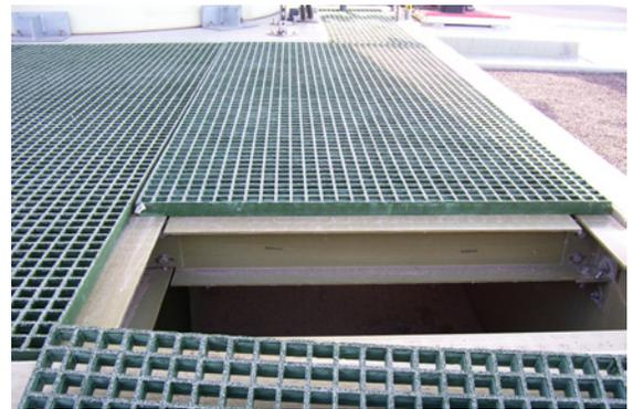
38.1mm DURAGRATE<sup>®</sup> was chosen along with EXTREN<sup>®</sup> wide flange beams as the support structure for a walking surface around equipment at a lift station that houses a wet scrubber for foul air treatment. DURAGRATE<sup>®</sup> has a high resin content (65%) which provides extended maintenance-free performance.
