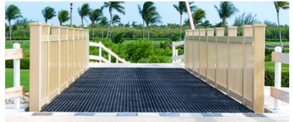
DURAGRATE® was chosen for this all-FRP bascule bridge because it could be outfitted with a grit system surface proving maximum traction while still remaining a non-marking walking surface, even in wet conditions. This 11.6m long, 3m wide Cayman Islands bridge is capable of supporting up to 2,268 kg.
