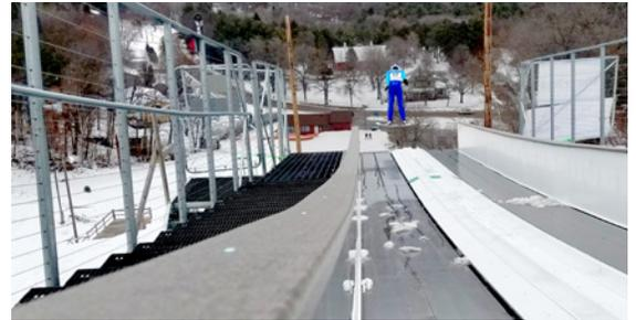
This 55-meter ski jump in Eau Claire, WI utilized DURAGRATE® molded grating and stair treads within the skier access and walking areas. Epoxy grit was applied to aid in long term slip resistance. DURAGRATE® allows for snow to melt or disperse through the grating, preventing excessive snow buildup which would have created slip hazards.
