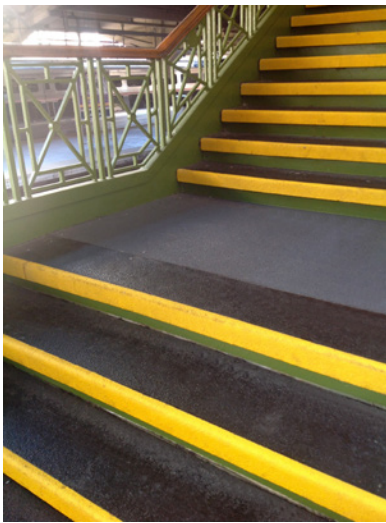
These rail station stairs in Baltimore, MD were renovated with DURATREAD™ stair tread covers, allowing the train station to keep the existing stairs, reduce downtime, and saver time and money in the process of the upgrade.
