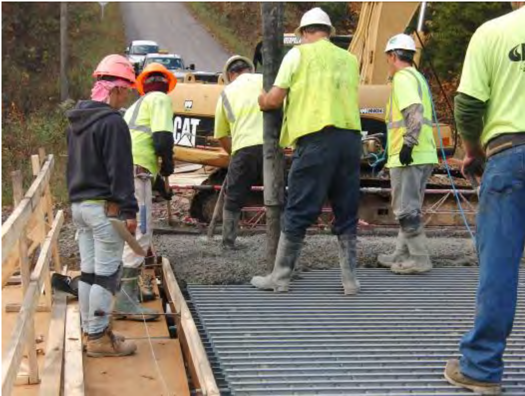
Figure 10. Concrete pouring and vibrating.
