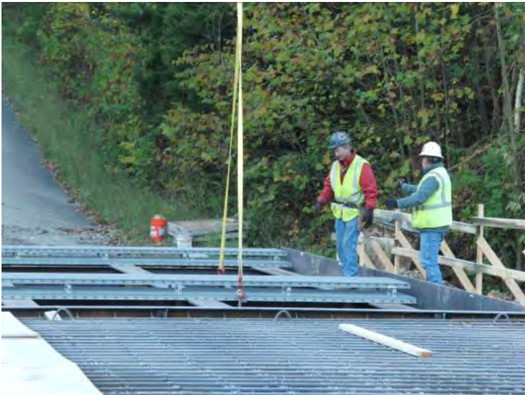
Figure 5. Placing FRP reinforcement panels by crane.
