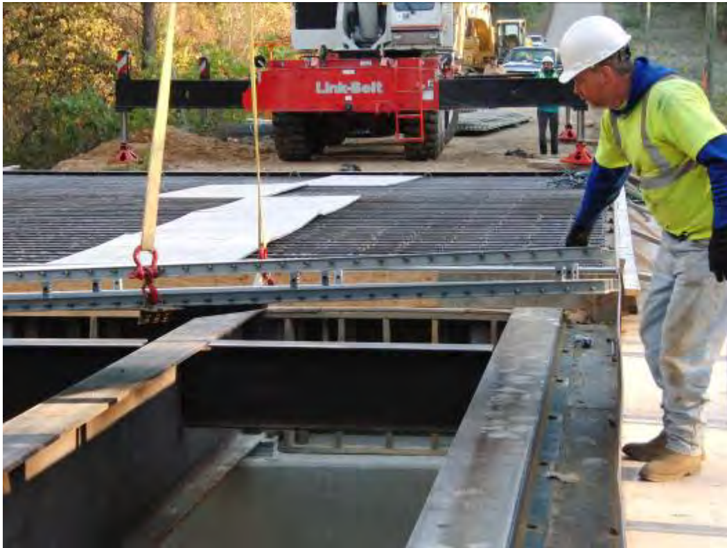
Figure 6. Guiding the FRP reinforcement panel installation.
