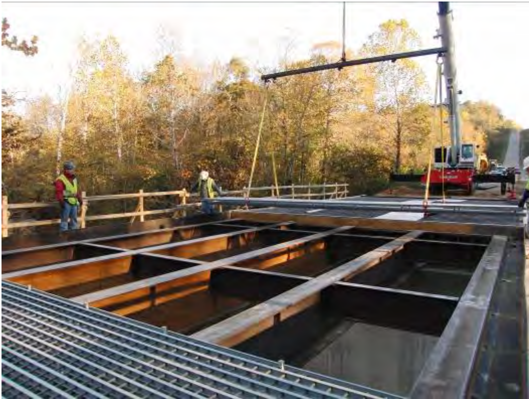
Figure 4. Crane lift of FRP reinforcement panels.
