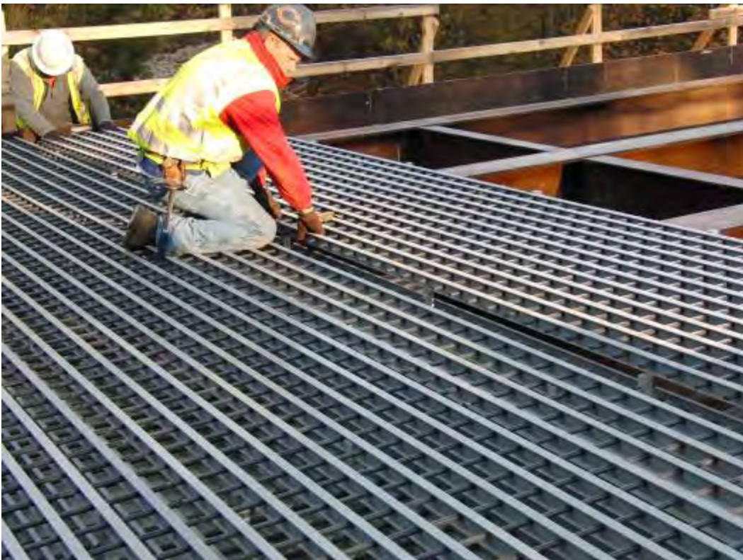
Figure 7. Manipulating the FRP reinforcement panels by hand.
