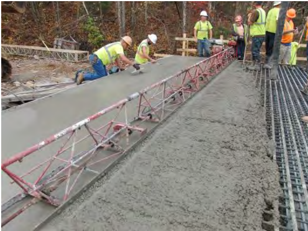
Figure 11. Spreading of concrete over the FRP reinforcement.
