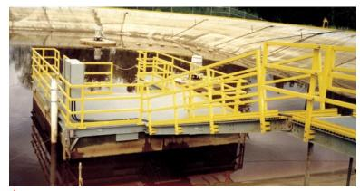
This floating dock uses lightweight, maintenance-free fiberglass handrail, flooring and structural supports.
