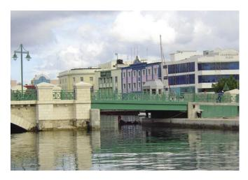
An all-composite double leaf bascule bridge recently installed in Bridgetown, Barbados, was built using Strongwell's COMPOSOLITE® building panel system, EXTREN® structural shapes and a custom heavyduty building panel. The bridge superstructure itself is made entirely of COMPOSOLITE® system components and custom building panels, while various sizes of EXTREN® square tubes were used to create an attractive architectural railing system.
