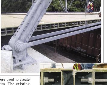
composite deck not only exceeds the life expectancy of the previous concrete deck but is also 70% lighter weight than a concrete deck. The deck allows the service load capacity of the bridge to be increased as well. The historic bridge will be completed by November 2006. ●
