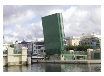
to-weight ratio of the pultruded parts. Heavier materials would have required the city to rebuild the lifting mechanism and other materials were not strong enough. The composite materials also offered the benefits of corrosion resistance, low maintenance and high aesthetic appeal.
