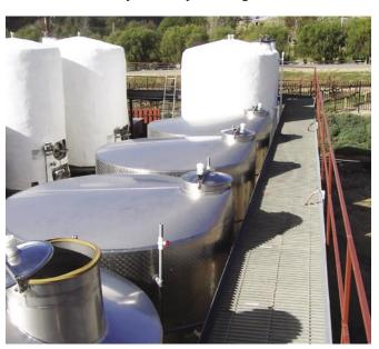
The new catwalk featured Strongwell's corrosion resistant DURAGRID® I-7000 1" pultruded fiberglass grating. Irvin International also used an EXTREN® 1" F-Track profile as kick plate.
