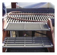
economical to ship and convenient to handle during installation. The fiberglass catwalk is also non-conductive and easy to maintain since the components will not require painting.
