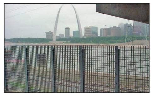
free fencing design using black and gray DURAGRATE® molded grating panels. Extra care was taken in choosing the material used in the county-wide project. Strongwell's black and gray DURAGRATE® molded grating was chosen because of its clean, attractive look, strength and corrosion resistance.
