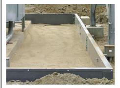
Chalk another one up for the timesaving COMPOSOLITE® Secondary Containment System! This type of containment is essential for substations. It is even mandated by the EPA because of the potential for oil leakage from transformers that may flow into adjacent bodies of water.
