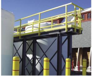
Therefore, it was necessary to build platforms using materials that were non-corrosive and safe.
