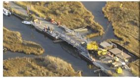
An FRP bridge deck by Strongwell solved logistics and maintenance problems by replacing a conventional wooden bridge deck on Tangier Island.
