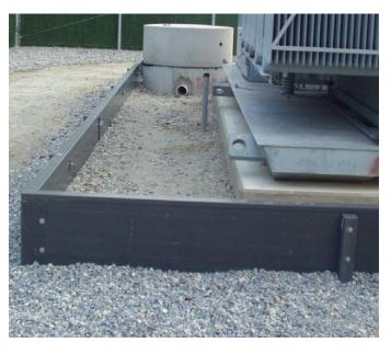
be easily removed if it becomes necessary to replace the equipment the containment systems surround. Added benefits of Strongwell's system include UV resistance, low thermal and electrical conductivity and a low maintenance life cycle.
