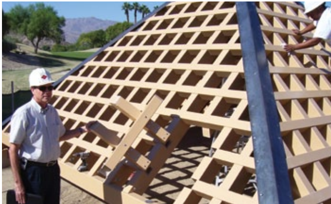
▲ David Kendall, project manager from Lee & Sakahara Architects AIA, in Irvine, CA, opens an access door to an assembled fiberglass pyramid prior to installation.
