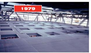
Anti-skid DURADEK<sup>®</sup> has always been known for excellent durability and the 30-plus year exposure on *Ellen* has had little to no effect on the grating. Even accidental sandblasting and paint overspray has not degraded the anti-skid surface. Previous reports indicated that abuse from the platform's SSV's (surface safety valves) and performing acid jobs have never been a problem. Workers experience less fatigue and a better kneeling environment with DURADEK<sup>®</sup> pultruded grating.
