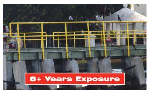
In 2002, Fort Lauderdale, Florida received the very first installation of Strongwell's round SAFRAIL<sup>™</sup> industrial handrail system below the city's 17th Street Bridge. The handrail was installed on the bridge's fenders.
