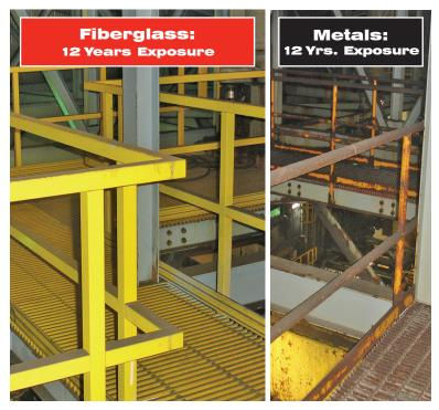
In 1994, Westfall Company teamed with the engineering group of Kerr McGee Coal Company to address corrosion problems at the Galatia, Illinois coal preparation plant. The coal preparation environment results in significant deterioration of carbon steel within two years and stainless steel in less than six. Kerr McGee's goal was to use as much non-metallic structural products as possible in the design of a new section of the plant.
