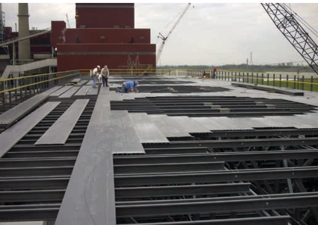
SAFDECK® is lightweight and easy to install, especially in rooftop applications like this cooling tower fan deck. The quick screw-down construction of the SAFDECK® system ensures rapid installation and reduced field labor costs.
