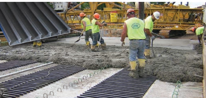
SAFPLANK®, when inverted, serves as an excellent concrete forming system in applications where corrosion and weight are construction concerns. Polyester resin is acceptable when pultruded FRP shapes are used as a stay in place (SIP) form. For concrete installations where long-term structural integrity is required, vinyl ester resin should be used.
