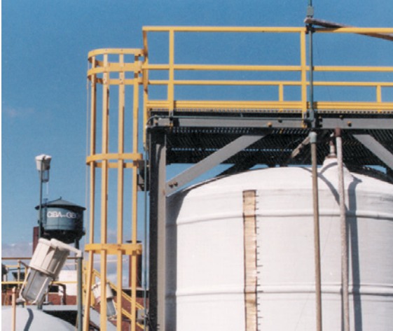
This fiberglass ladder and cage provide worker access to a maintenance platform at a Ciba Geigy plant in the northeastern United States.
