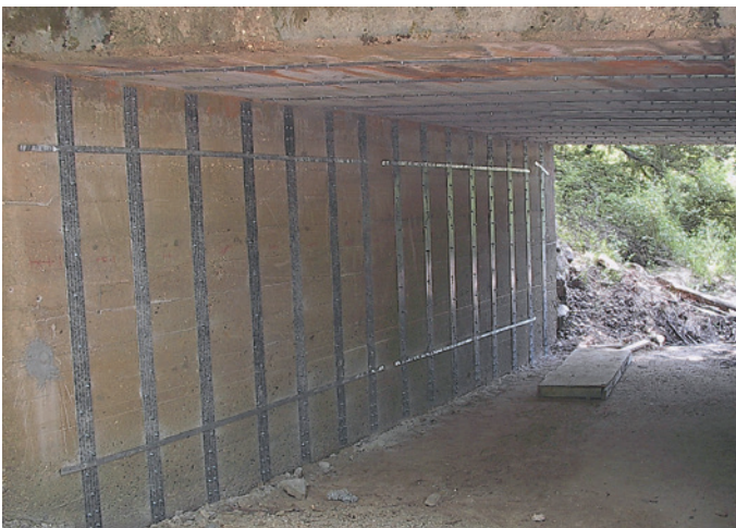
The abutment and deck of this bridge in Phelps County, Missouri, was strengthened using SAFSTRIP®. As a result, the existing 12-ton load posting was removed.
