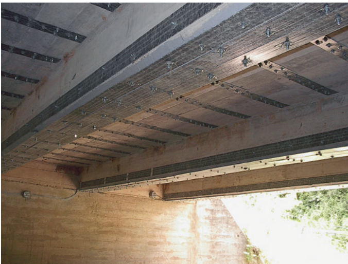
The posted load for this bridge that spans the Meramec River in Missouri was increased from 10 tons to 18 tons by installing SAFSTRIP® using the MF-FRP system.
