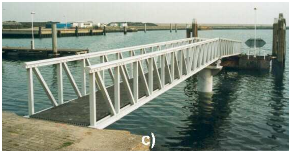
Fig. 7. Noordland pedestrian bridge: a) ready for shipment; b) installation; c) in service.
