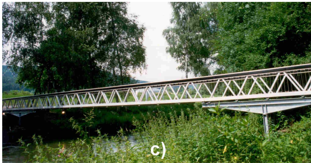
Fig. 3. a) Stainless steel bridge in Den Bosch, the Netherlands; b) FGRP bridge near Łódź in Poland (courtesy Fiberline Composites A/S); c) Aluminum bridge near Böblingen, Germany (courtesy PML Logis-Systembrücke).
