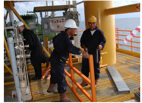
Orange SAFRIL™ being field fabricated by factory trained installers in the South China Sea. Square tube handrails are easily field fabricated, however, round tube handrail is more difficult and should be fabricated in a qualified shop.
