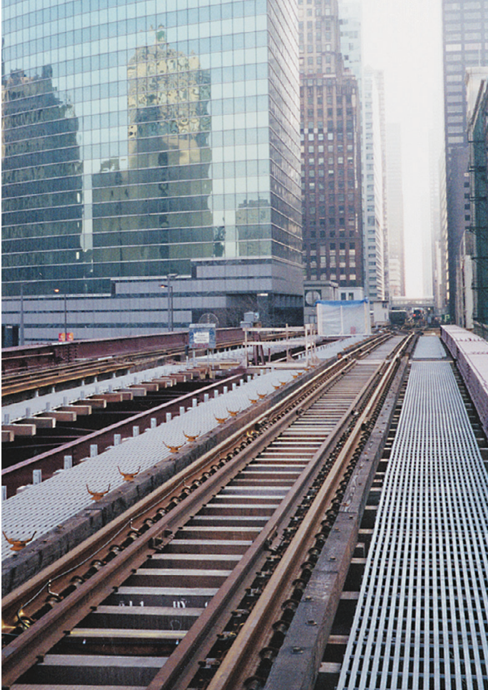
Chicago Transit maintenance walkways alongside elevated train tracks constitute one of the largest fiberglass grating installations in history. This project used T-5000 51mm with a custom polyester resin.
