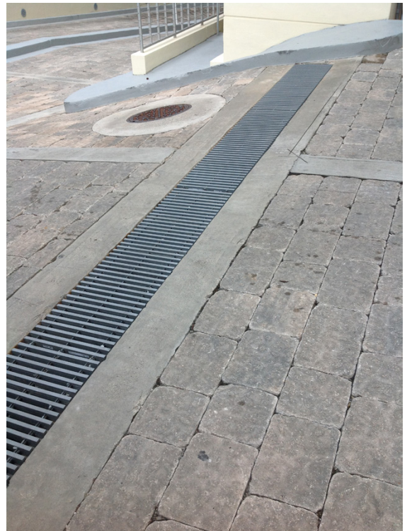
HD-5000 38mm was used at a high-end condominium complex in Miami Beach, Florida to cover drainage channels at parking garage entryways.
