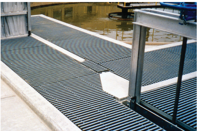
Low maintenance fiberglass grating provides trouble free operations for the covers and walkways in the Lakewood, Colorado Wastewater Treatment Plant Headworks. I-6000 38mm was used.
