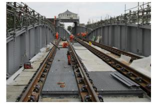
and was well in need of a refurbishment for steelwork, hydraulics, beams, and paint. With a budget of over \$10 MM dollars, the owner and operator of this bridge had to consider factors such as weight, historical preservation, durability, electrical conductivity, and corrosion resistance in all of its materials.
