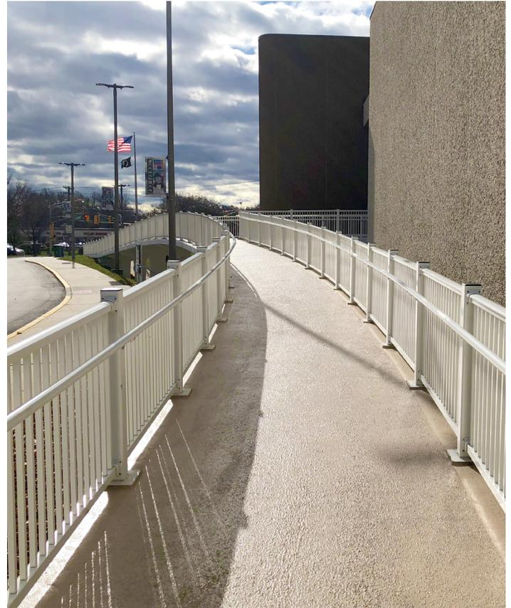
The installers were happy with the simplicity of the field fabrication of over 600 linear feet of STRONGRAIL®, with its internal connection system. In their opinion, the handling and installation process was much simpler, compared to traditional steel. With no hot works or specialty steel fabrication crews required, installation was faster, easier, and less expensive than steel, and should provide years of low- to no-maintenance performance. ●
