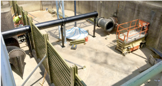
This wastewater treatment facility in Ohio installed Strongwell baffle panels along with EXTREN® wide flange beams, square tubes, and angles, which enabled each chamber to generate higher biomass solids concentration resulting in better bio-treatment.
