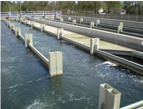
Above: Keegan's Bayou Wastewater Treatment Plant in Houston, TX, installed this baffle system in 2002. This system was selected over traditional materials (aluminum, stainless steel, poured-in-place concrete, and concrete columns with redwood baffles) due to extended product life cycles, especially in highly corrosive chlorine contact chambers.
