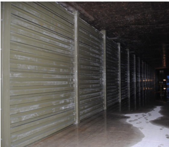
The Lima, OH, Waste Water Treatment Plant required an underground baffle system to allow the water to move more slowly, resulting in better primary sedimentation. This installation was accomplished without the use of cranes or any other lifting equipment due to the lightweight panels and structural members used.
