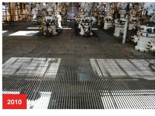
With over 40 years of daily exposure to weather and pedestrian traffic, the grating still retained over 80% of its flexural modulus and 80% of its maximum load capability from its published load tables. As tested against the published data
