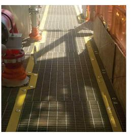
In this particular case study, Strongwell's custom phenolic plate was integrated within a steel grating flooring system on an offshore
