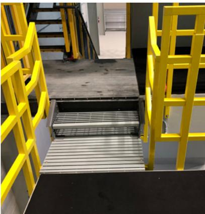
On each of the landings, T-1800 DURAGRID® pultruded grating panels were chosen due to span, weight, and open space guidelines. This particular series of T-shaped bar grating offers 18 percent open space while weighing only 2.6 lbs. per square foot.
