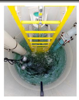
Manufactured by Strongwell in the USA since the 1950s, fiberglass ladders have demonstrated outstanding durability in complete fluid immersion applications versus steel and aluminum.
