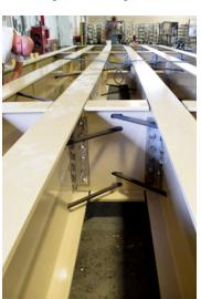
fully utilize EXTREN® Series 625 square tubes and wide flanges to construct the pedestrian handrails and pickets. The supporting structure of this bridge took advantage of FIBREBOLT® to mechanically fasten EXTREN® angles, tubes, I-beams, and wide flanges together.
