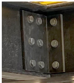
FRP Double clip angle connection
