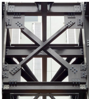
FRP Gusset plate connection
