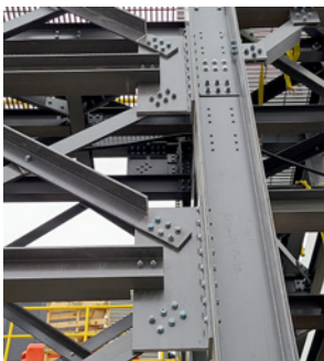
FRP WT-Shape connection
