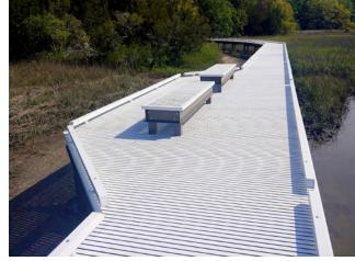
used. Square tubes, channels, plates, and I-beams were fabricated for seating areas and to support the entire walking surface of the boardwalk.
