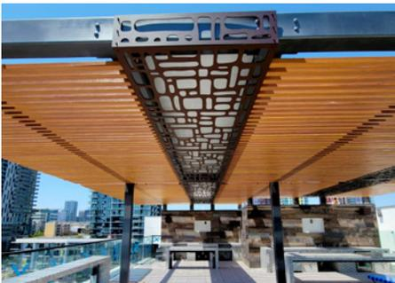
Each of the 6"x 9" tubes were coated with metallic paint to produce a custom finish.
