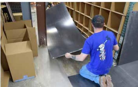
Over a period of two days, a three-member contractor team was able to lay out, fabricate, and adhere all of the flat sheet panels via silicone adhesive throughout the distribution area.
