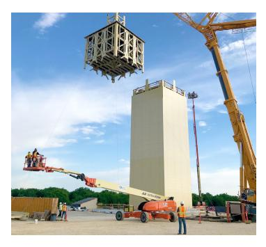
Over 28,000 FRP threaded hex nuts, 13,400 linear feet of threaded rods, and almost 30,000 linear feet of DURASHIELD® was used for exterior cladding. The weight of those three items totaled almost 260,000 lbs, of composites.
