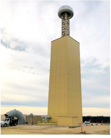
The end user reported that they were pleased with the project timeline and material performance. The structure was erected onsite in phases due to internal access and safety structures (handrail, ladders, cages, and landings) being simultaneously installed. Weight reduction played a major role as each fabricated section had to be hoisted, stacked, and fastened to one another.
