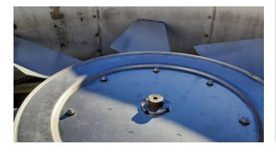
Prior to launch, this custom pultruded profile endured thousands of hours of product testing to ensure the blades were capable of enduring high cycles of fatigue throughout a wide range of temperatures. In these temperature tests, temperatures reached up to 180 degrees F.
