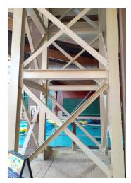
All five landings and accompanying stair treads were outfitted with 1" DURAGRID® T-1800 panels with 18% open space ensuring water flow and light allowance. Panels were coated with slip-resistant grit safe for bare feet.
