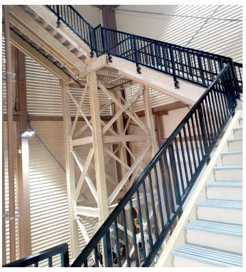
All mechanical connections were secured with stainless steel hardware as an added preventative corrosion measure.
